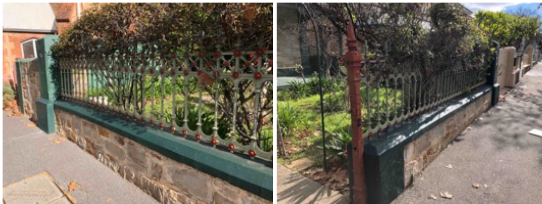
Figure 44 Front wall to be conserved Source: Flightpath Architects, July 2018.
