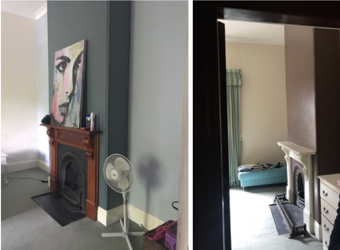
Figure 17 Chimneys within the bedrooms upstairs: note non-original cornice Source: Alexander Brown Architects, 2017.
