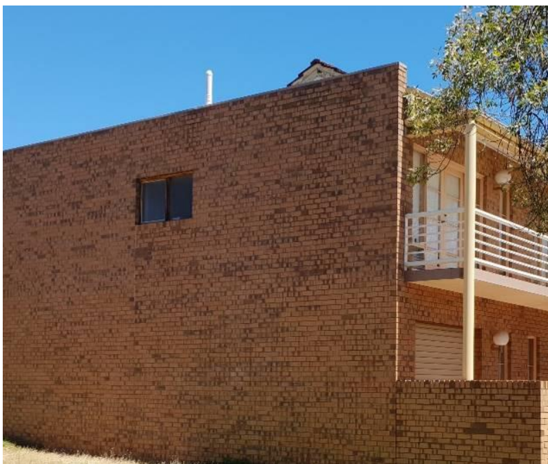
Figure 2 – Existing upper level window on eastern façade of neighbouring dwelling to the west (227 Childers Street)
