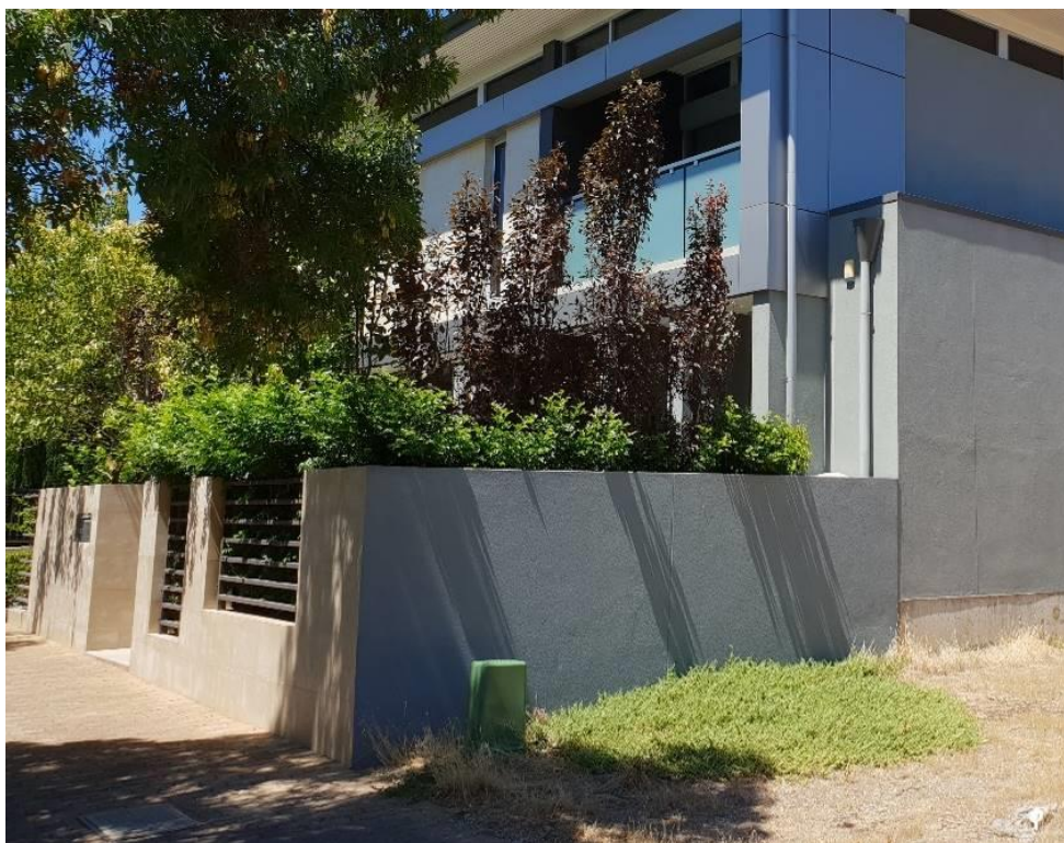
Figure 3 – Existing wall and landscaping located adjacent boundary of eastern dwelling (223 Childers Street)
