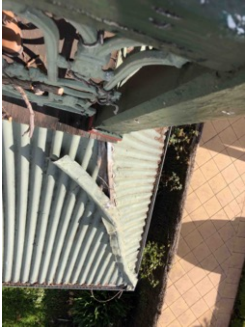
Figure 39 Balcony Dilapidation Source: Flightpath Architects, 2018.
