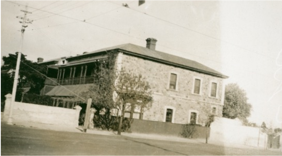
Figure 9 Adjacent buildings, 1934 Source: State Library of South Australia.
